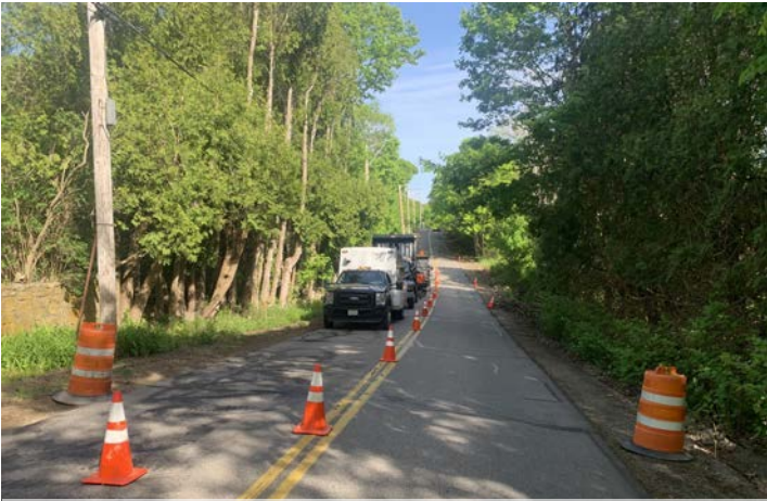
Work on Southside Road.
