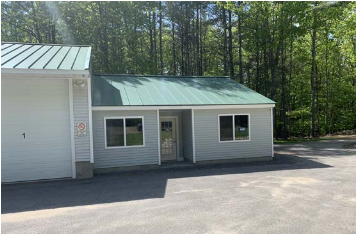
Progress on the RPO renovations.
