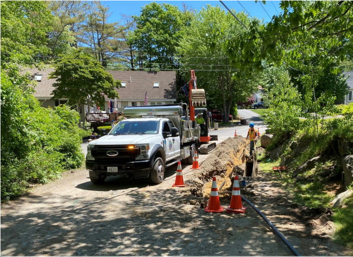
New Pipe on Nicole Road
